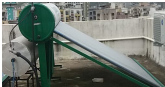
500 LPD Solar Water Heater
