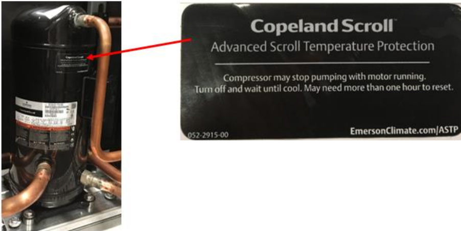
Figure 13: Advanced Scroll Temperature Protection (ASTP)
