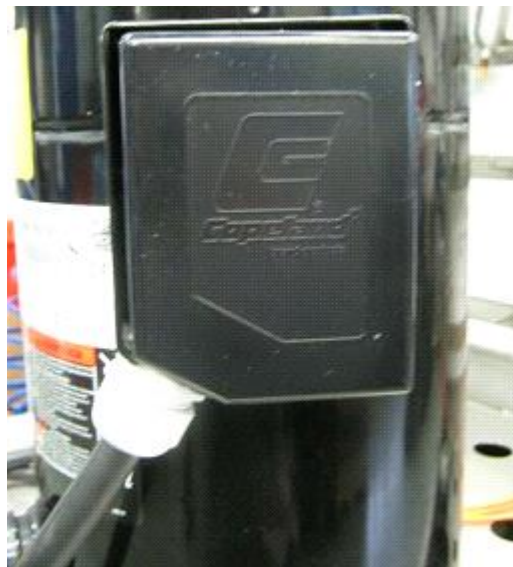
Figure 20: Correct electrical installation with cable glands for IP21 T-box, models ZR108KRE to ZR190KRE
