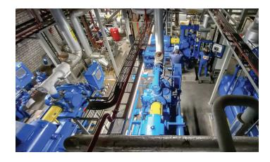
The system still uses the original four Vilter ammonia compressors on its high side. For added reliability and continuity during scheduled maintenance, the system was designed to repurpose the previous reciprocating  $\mathrm{CO}_2$  compressors in a backup role.
