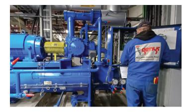
Because of its higher capacity, one Vilter  $CO_2$  single screw compressor replaced the existing two reciprocating  $CO_2$  compressors. In fact, the cooling capacity of a  $CO_2$  single screw compressor is 830 kW at -40 °C (-40 °F) evaporation and -7 °C (19 °F) condensation temperatures — nearly doubling the capacity of its predecessors. Ideal for subcritical  $CO_2$  applications, the Vilter  $CO_2$  single screw compressor now serves as a reliable anchor for the low side of the system.
