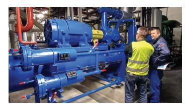
The culprit of a persistent maintenance problem was an oil carry-over issue in the reciprocating CO<sub>2</sub> compressors. But even after taking steps to mitigate this, the reciprocating compressors required excessive maintenance. The system
