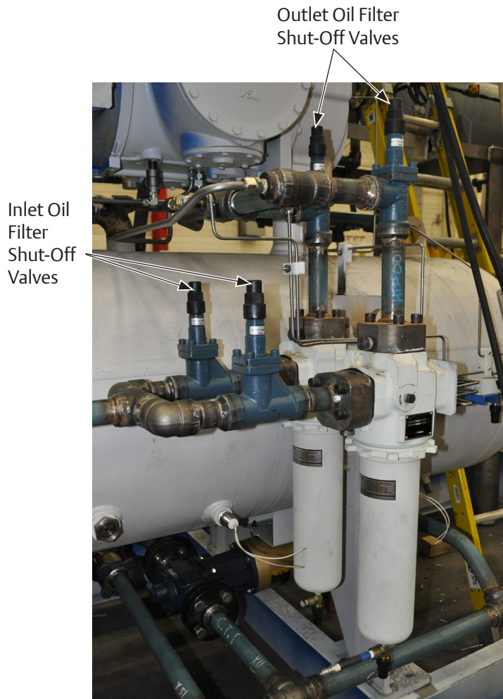
Figure 4-9. Dual Oil Filter Setup for Oil Filters with Manifold Heads
