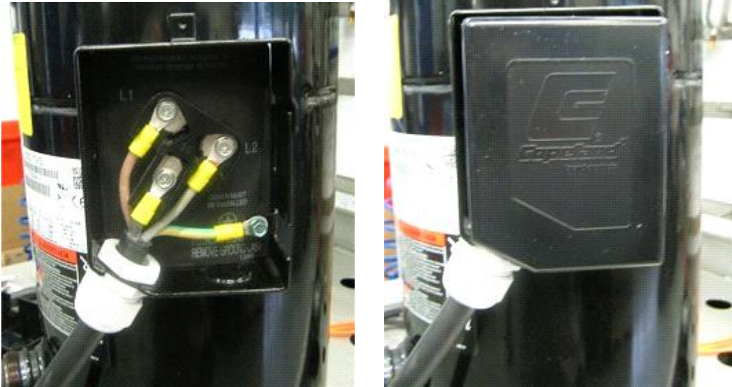
Figure 14: Terminal box IP21 and correct electrical installation with cable glands
