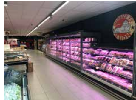
Medium temperature cabinets from Delhaize store, equipped with the Copeland ZX A2L refrigeration unit.
