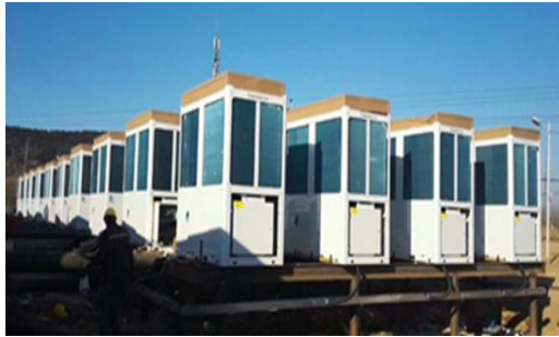
A district heating project in Beijing
