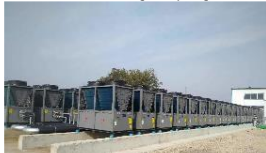
Heating project in a residential building in Shandong
